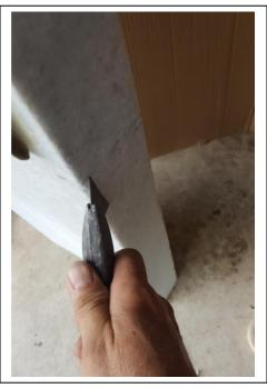
**Step 9**. Clean the headstone where the excess got on the surface of the headstone. I used automotive grade lacquer thinner very lightly. It cleans fast and evaporates faster. Denatured alcohol can be used also. I had to clean out excess epoxy from a few of the numbers in the death date but if you do it early it isn't a problem to do. As you can see, the fix is almost invisible up close. From 20 feet away it is invisible.
